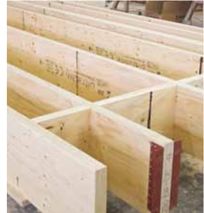
Pre-assembled box girders for roof construction.
